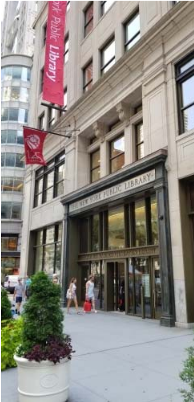
Exterior of newly renovated Stavros Niarchos Foundation Library (SNFL). It was formerly the Mid-Manhattan branch and prior to that, a department store. Adaptive re-use!
