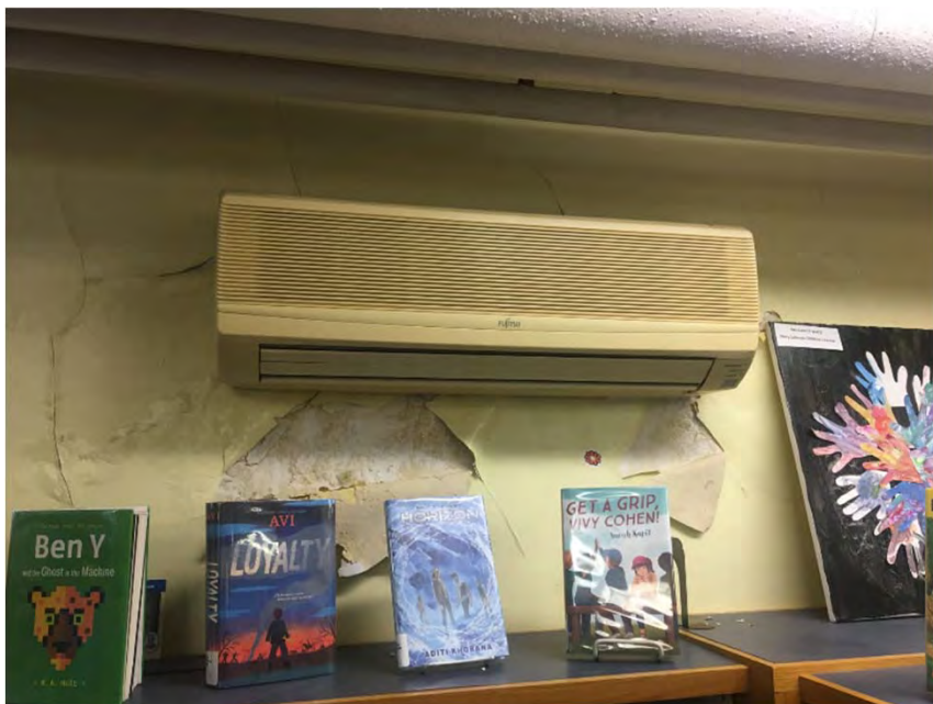
An AC unit that is so old the parts are no longer available for servicing.
